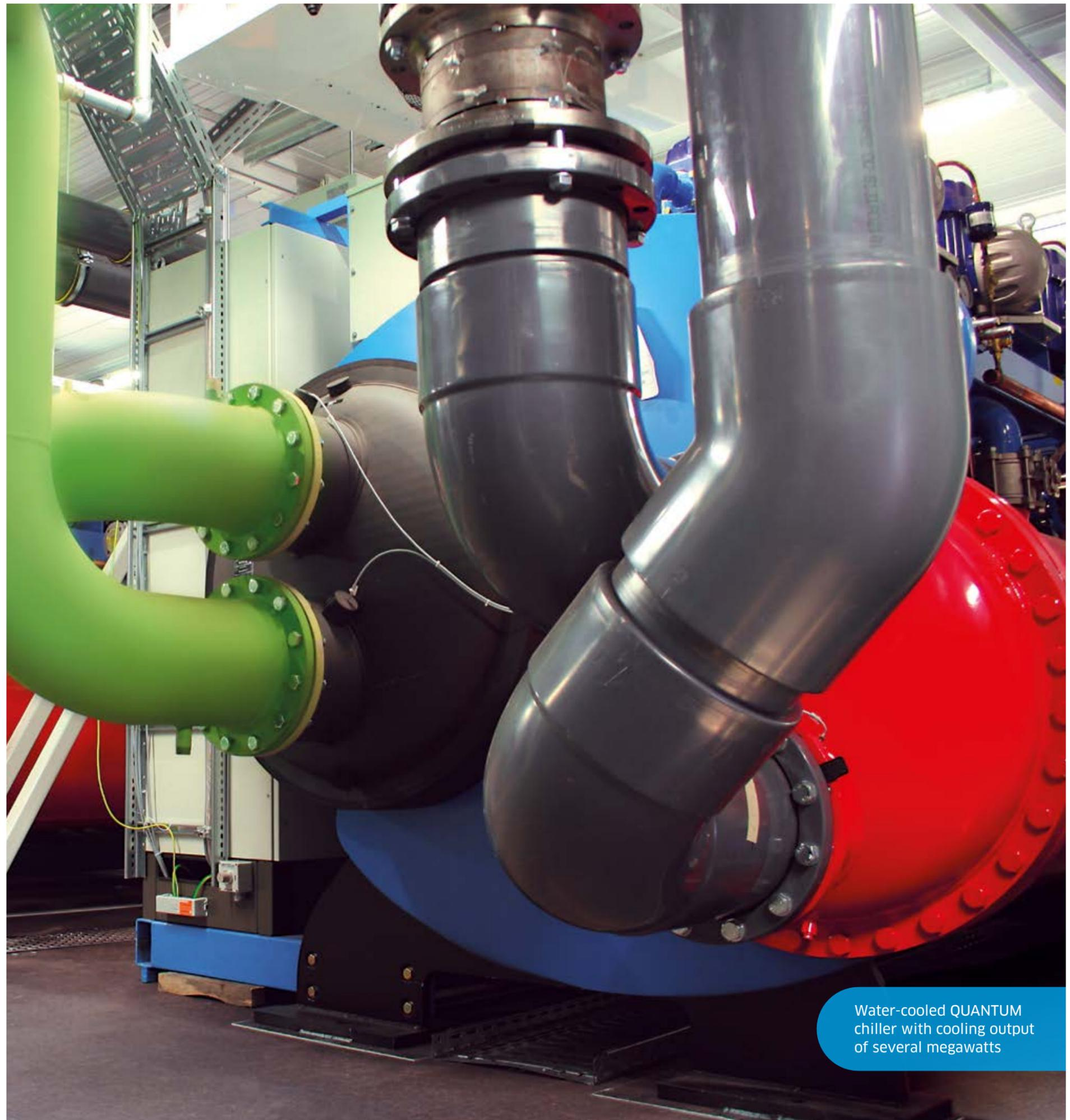
Water-cooled QUANTUM chiller with cooling output of several megawatts
