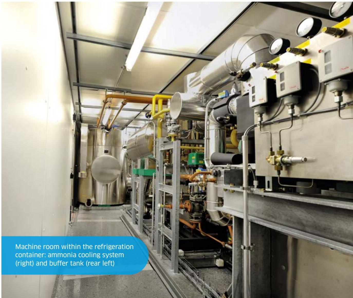
Machine room within the refrigeration container: ammonia cooling system (right) and buffer tank (rear left)
